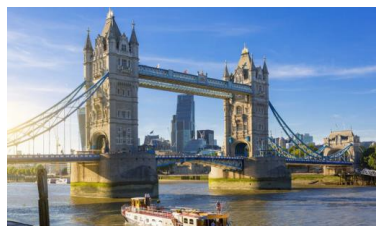
Figuur 8. Tower Bridge
